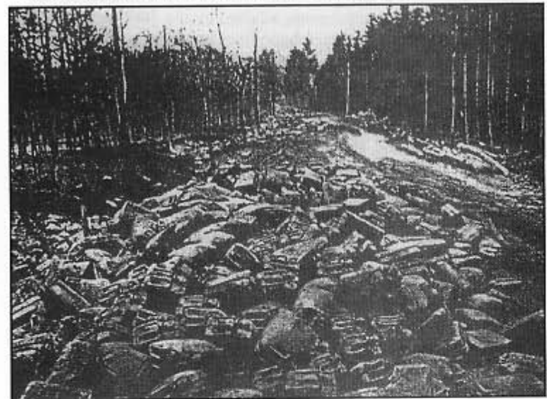
The job when they finished.
